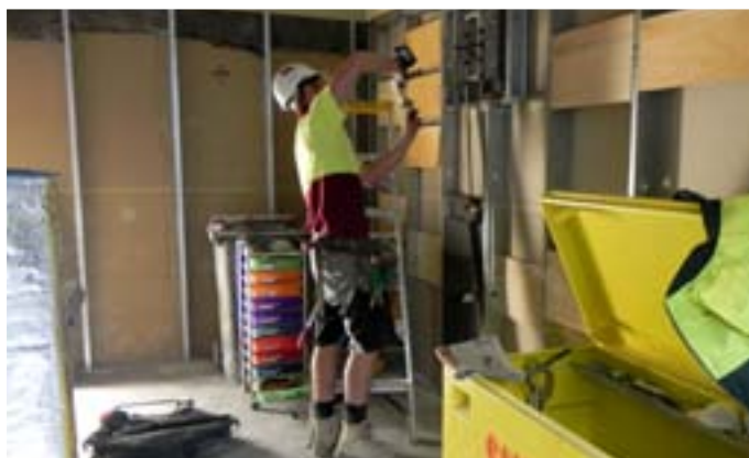
Sanwell Plumbing have over 70 plumbers onsite
